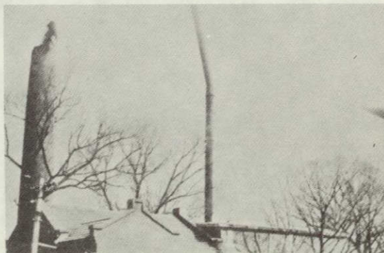
Photo 10: The top 7-8m of the 27m tall brick chimney of the boiler of Tangkangtze Sanatorium in Anshan City was knocked off, while another iron chimney was bent in the direction of 310° northwest. (Mag 7 area)
