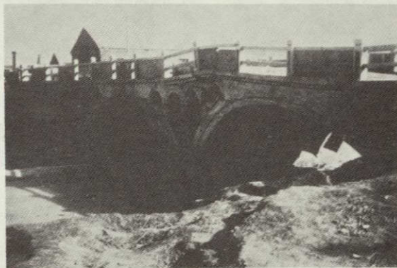
Photo 8: The mid-section of Hungkwang Great Bridge in Kwenchipao of Chikao Commune in Yinkao Prefecture, buckled and the arch was destroyed after the quake. (Mag 8 area)
