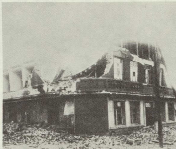
Photo 6: Collapsed parts of walls and roofs of brick and wooden buildings on the corner of 5th street and People's Road, Tiehsi, Anshan City. (Mag 7 area)
