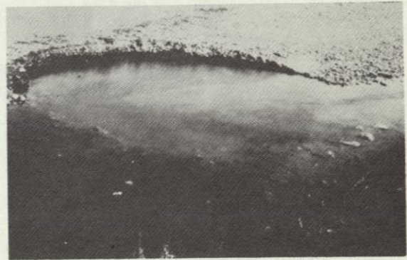
Photo 26: Depression in the river bed north of Koshan Commune, Haicheng. The wall of this hole consists of loose gravel. According to a report, the depth of depression was 4m, and the diameter of the crescent shaped depression was 5m. (Mag 8 area)
