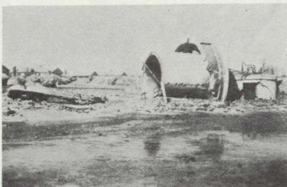
Photo 11: The inverted water tank (29.5m tall) in East Family District of Senseng Farm, Yingkao Prefecture, toppled over. (Mag 8 area)
