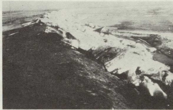
Photo 18: Approximately 1m thick ice on Yungshung Dam in Panchin district was pushed up onto the embankment. There were cracks in the ice along the edge of the dam caused by pressure. (Mag 7 area)
