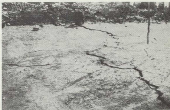
Photo 14: The brick wall of Kuh Fang-sen Hosi Elementary School of Punkao Commune, Haicheng Roof slates collapsed after the quake. There were two sets of cracks in the earth, one set running north-south, the other east-west. Width 5-15cm, visible depth 1.35m. (Mag 9 area)
