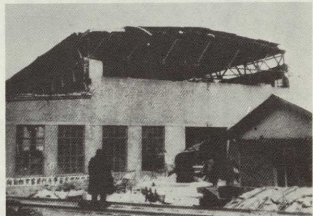
Figure 14: Collapsed walls on the ends of a building
