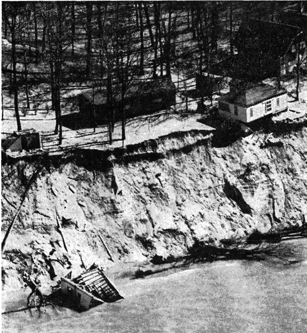
Lake Michigan Cottage Near Palisades Park Has Fallen In Water
