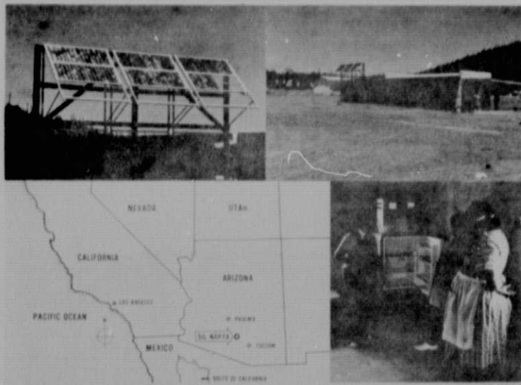
Figure 1. - Photovoltaic powered refrigerator. At Papago Indian Village of Sil Nakya, Arizona.
