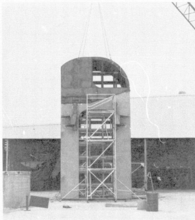
Figure 7. Completely Fabricated Blast Structure, TSM Prototype
