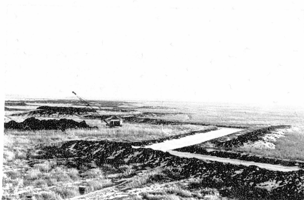
Figure 5. Photograph illustrating level ditch construction.
