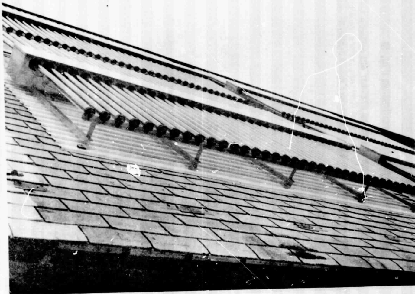
Figure 7. Collector array reflective backing. White vinyl siding used on MSFC Solar Demonstration Facility, Huntsville, Alabama.
