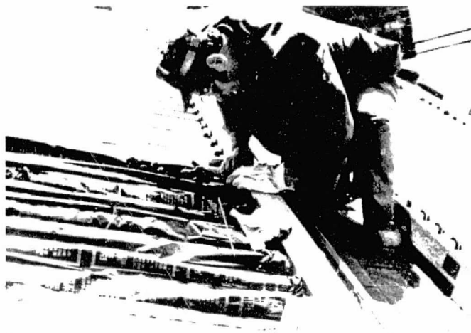
Figure 5-2. Firmly Seat Grommet into the Collector
