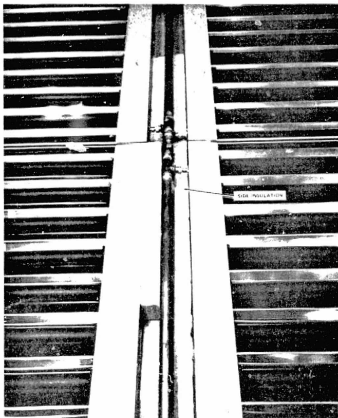
Figure 5-10. Insert Insulation Around Header Pipes
