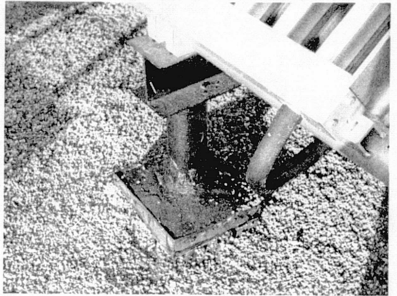
INSULATION PRIOR TO COATING
