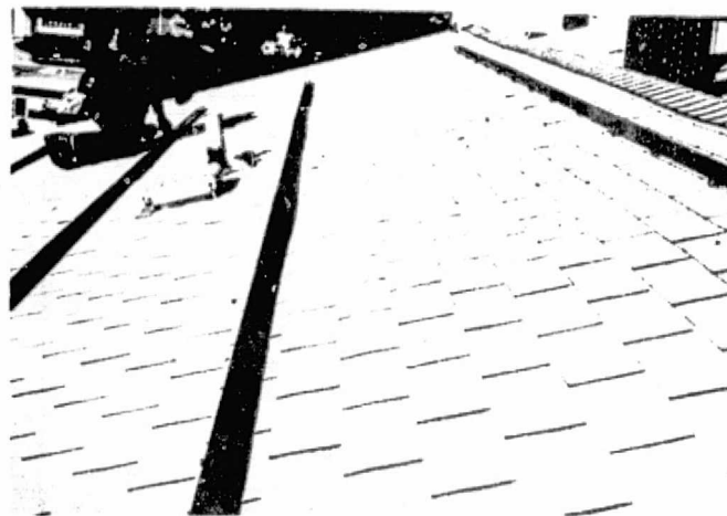
Figure 3-10. Attach UNISTRUT to Roof
