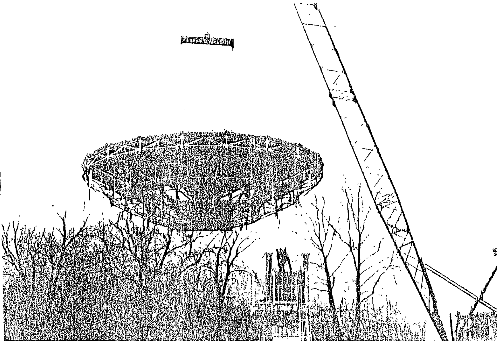
FIGURE 67. TYPICAL REFLECTOR STRUCTURE/PANEL ASSEMBLY BEING LIFTED
