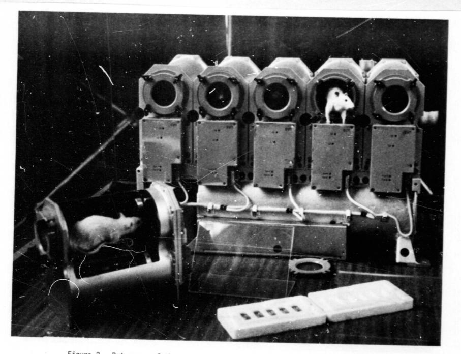
Figure 2. Rat cages of the type flown on Cosmos 1129. Cages are placed aboard the spacecraft in blocks of five cages. The cages in a block share food and water reservoirs.
