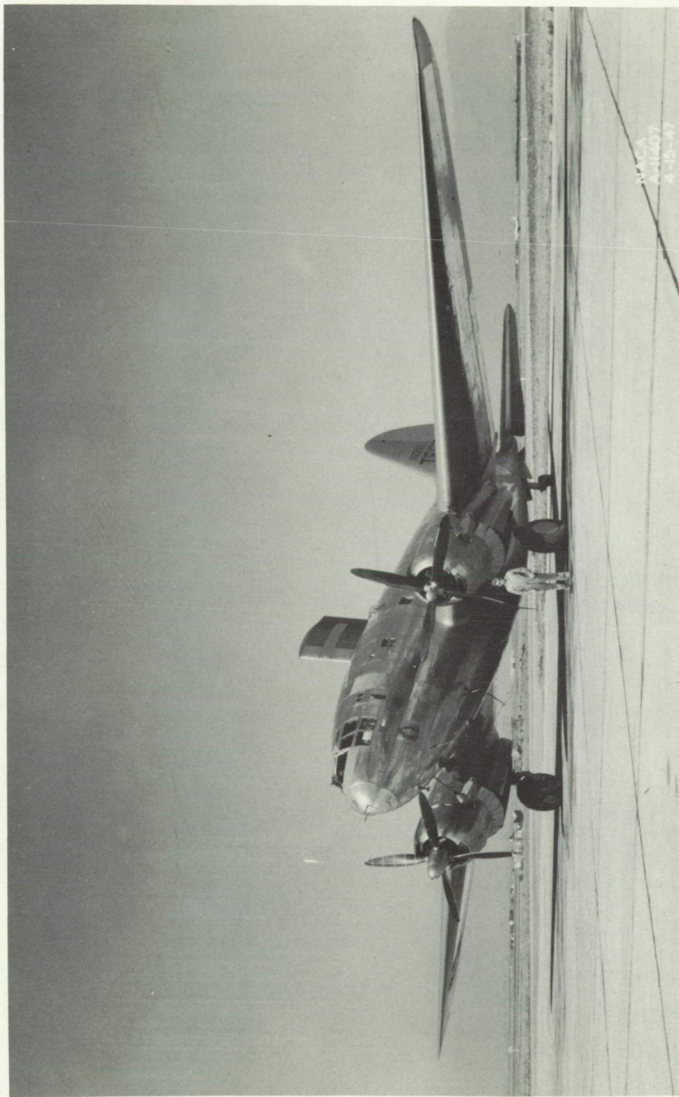
Figure 2.- The C-46 airplane as equipped for icing research flights in the winter 1946-47.
