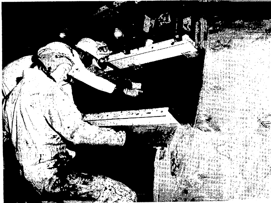
Figure 27.- Installation of internal insulation.
