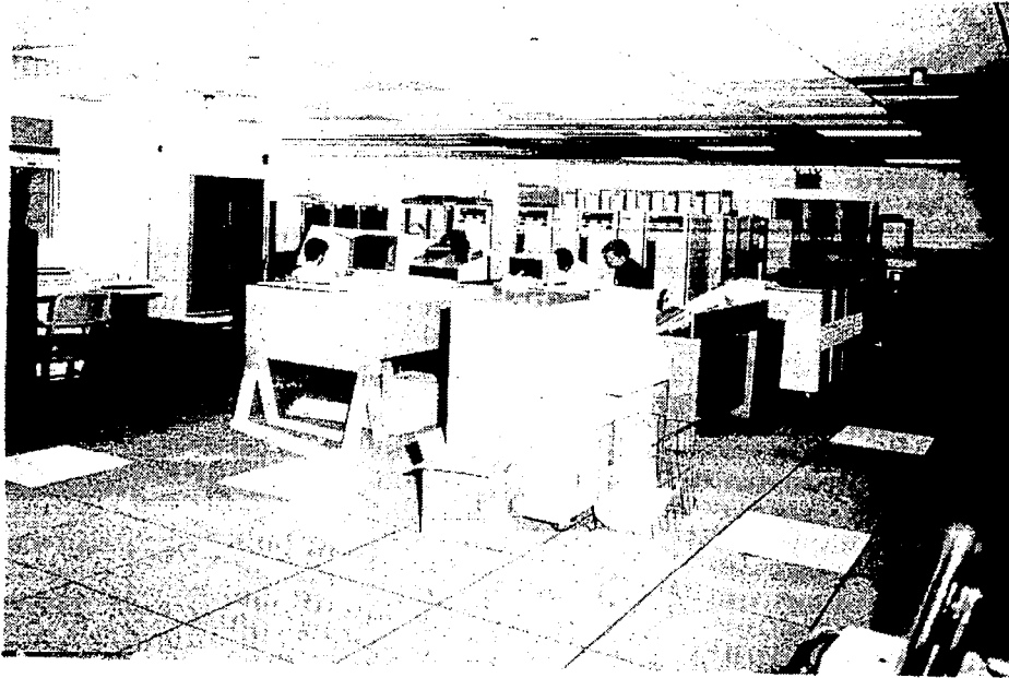
Figure 37.- Photograph of control room showing computer system.
