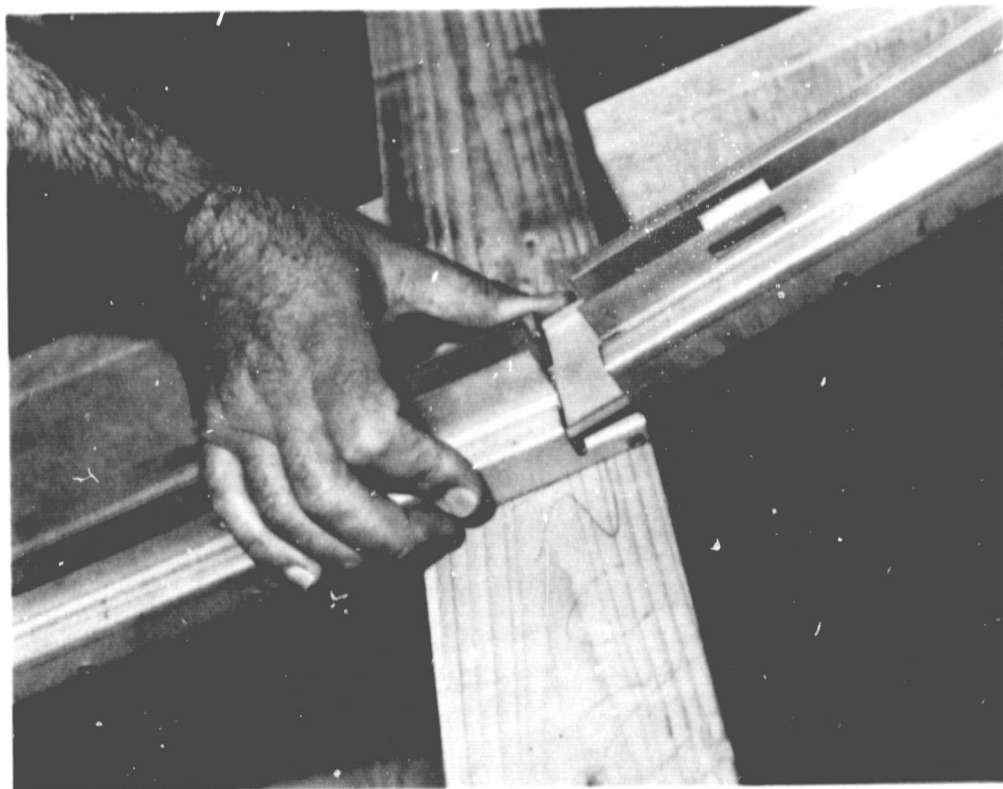
Figure 3-44. Installation of Support Channels
