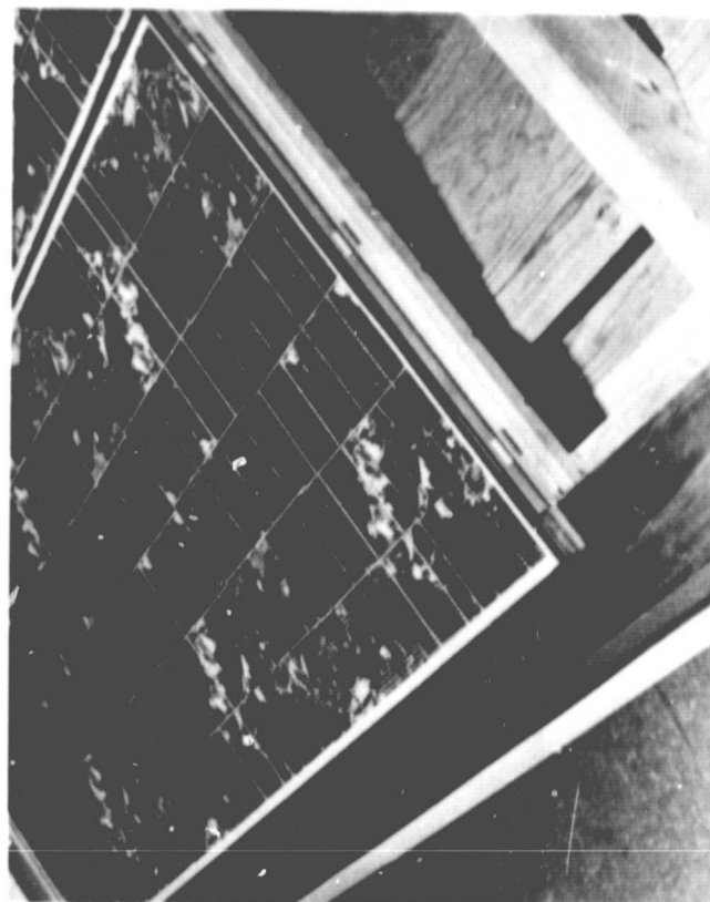
Figure 3-4 c Module Interface with Support Hardware at Eave and Rake
