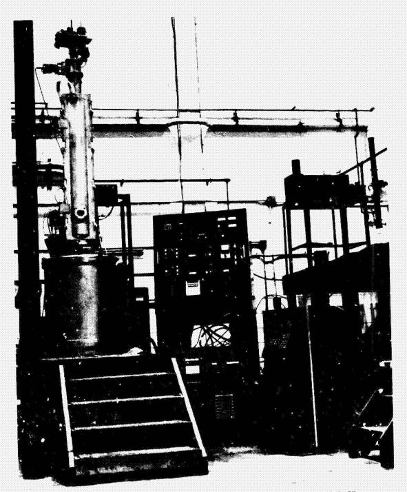
THIS IS A PHOTOGRAPH OF THE FIRST CG6000 WHEN IT WAS BEING ASSEMBLED. THIS MACHINE WAS PURCHASED SPECIFICALLY FOR SOLAR INGOT PRODUCTION USING THE JPL-DEVELOPED PERIODIC RECHARGE METHOD. IT IS PLANNED TO PRODUCE 60 TO 80 KILDGRAMS FROM EACH CRUCIBLE. ALTHOUGH THIS IS NOT THE QUANTITY DEEMED TO BE THE MOST COST EFFECTIVE, IT IS CERTAINLY A MAJOR STEP TOWARD LOWER COST SOLAR GRADL MATERIAL.
