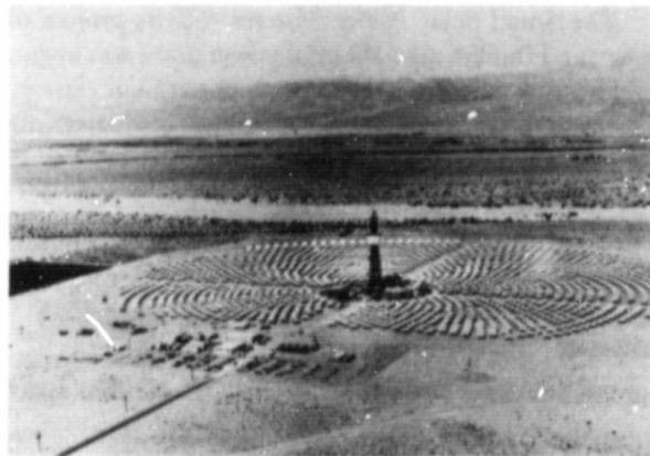
Figure 2-14. Completed Collector Field at Barstow Pilot Plant, September 1981
