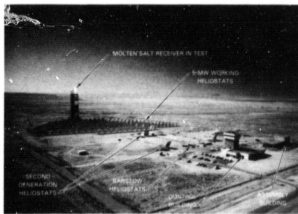
Figure 2-30. 5-MWe Central Receiver Test Facility
