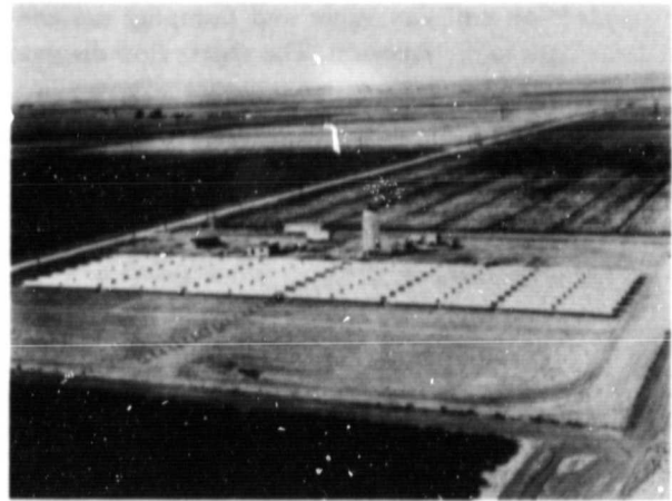
Figure 4-14. Deep-Well Irrigation Project, Coolidge, Arizona
