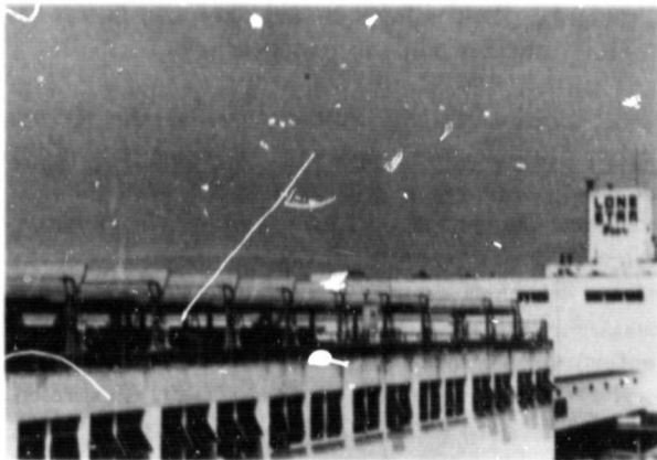
Figure 4-18. Collectors in Operation at Lone Star Brewery
