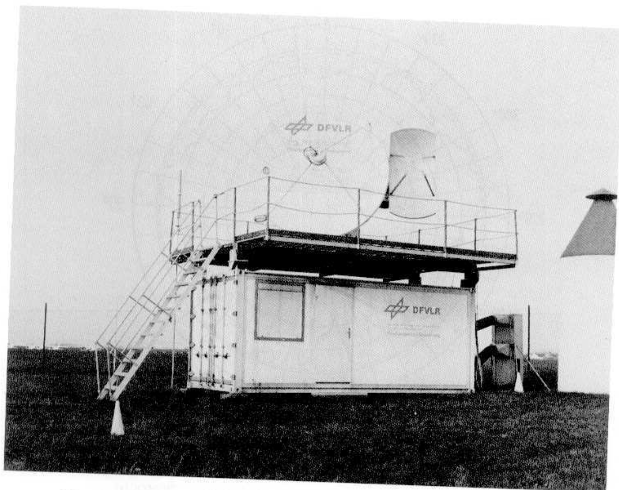
Fig. 5: Ground Station Container and Antenna Systems
