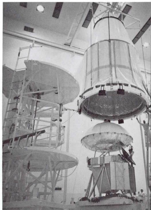
Viking orbiter 1, top left, is mated to Viking lander 1 at Kennedy Space Center on 8 March 1975. Above, technicians lower the launch shroud over the spacecraft on 27 March. At left, the shrouded orbiter and lander move toward 31 March mating with the Titan IIIE launch vehicle, for more tests.
