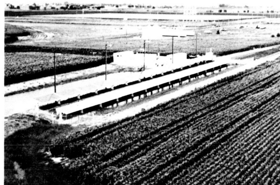
A 28-kW array of solar cells for crop irrigation during summer, and crop drying during winter (a DOE/University of Nebraska cooperative project).
