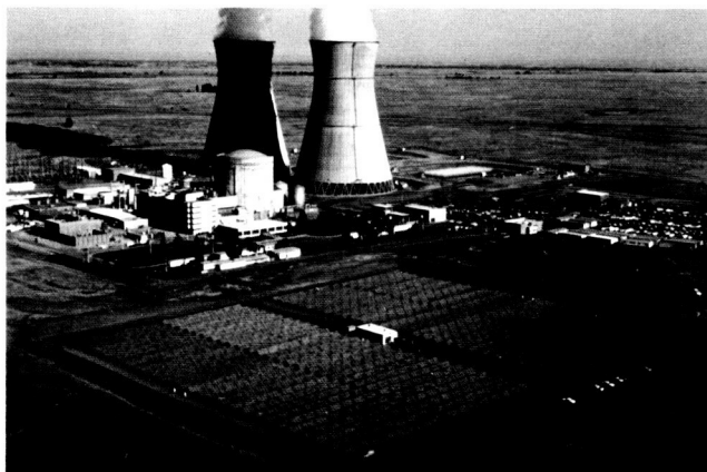
1.2 MW of photovoltaic peaking-power generation capacity for the Sacramento Municipal Utility District. (The 8 x 16 ft panels are mounted on a north-south axis for tracking the sun.)
