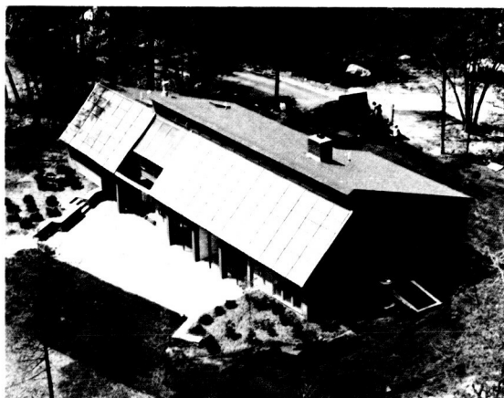
House in Carlisle, Massachusetts, with a 7.3-kW photovoltaic rooftop array. Excess photovoltaic-generated power is sold to the utility. Power is automatically supplied by the utility as needed.
