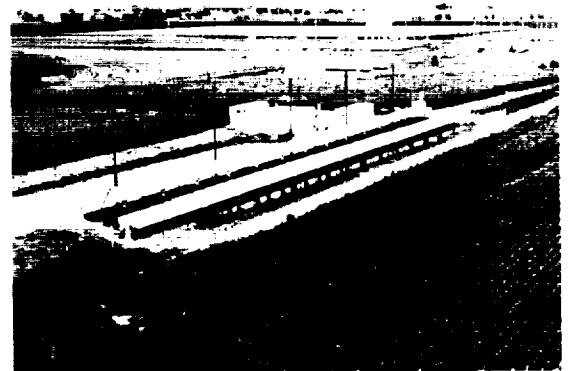
A 28-kW array of solar cells for crop irrigation during summer, and crop drying during winter (a DOE/University of Nebraska cooperative project).
