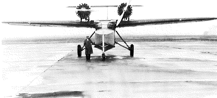
This twin-engine Douglas Dolphin amphibian was unusual in that it employed a nose wheel instead of a tail wheel, January 1937.
