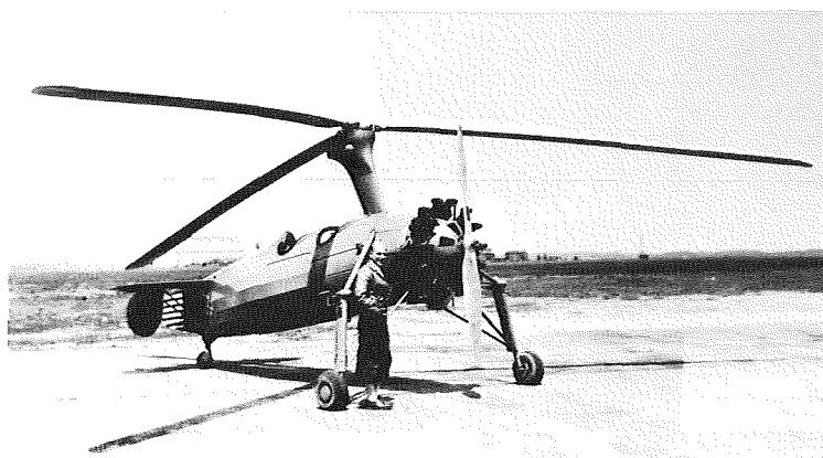
Kellett autogiro, April 1936. This type of aircraft could make extremely short takeoffs and landings, but it was not capable of the helicopter's hovering or vertical flight. In theory the autogiro's main advantage over the conventional airplane was that, in the event of engine failure, its autorotation permitted safe descent.
