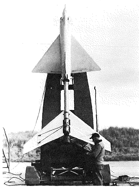
At Wallops Island in 1953, Langley's Pilotless Aircraft Research Division (PARC) tested rocket-powered models of the delta-winged Convair F-102 before (left) and after (right) application of the area rule.
