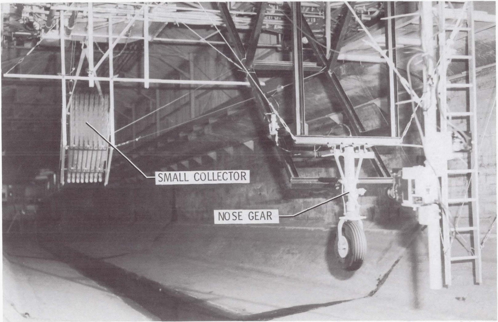
Figure 7. View of water-collector array and nose gear mounted on test carriage.
