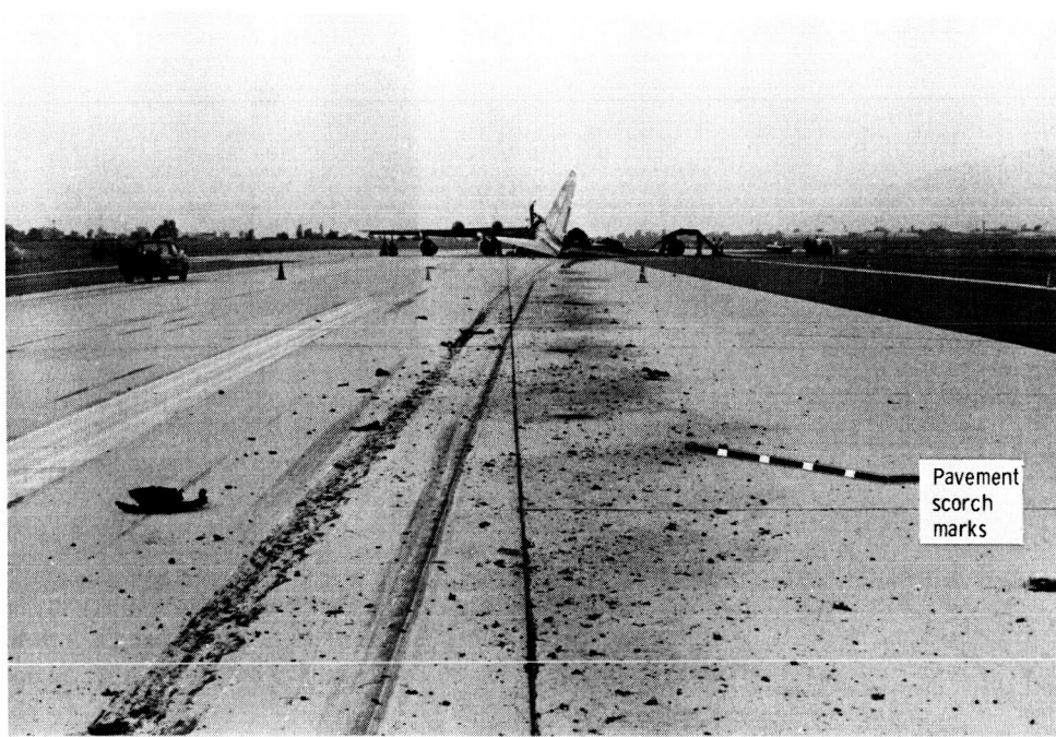
Figure 10. - Runway surface scorch marks and tire rubber debris from right main gear at about 11,950 ft down runway 32.
