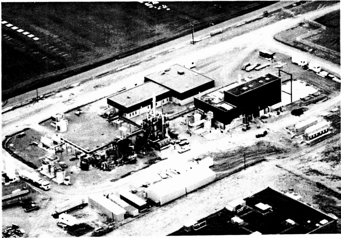
Figure 5. A 100-MT Silane Process Pilot Plant, Washougal, Washington
