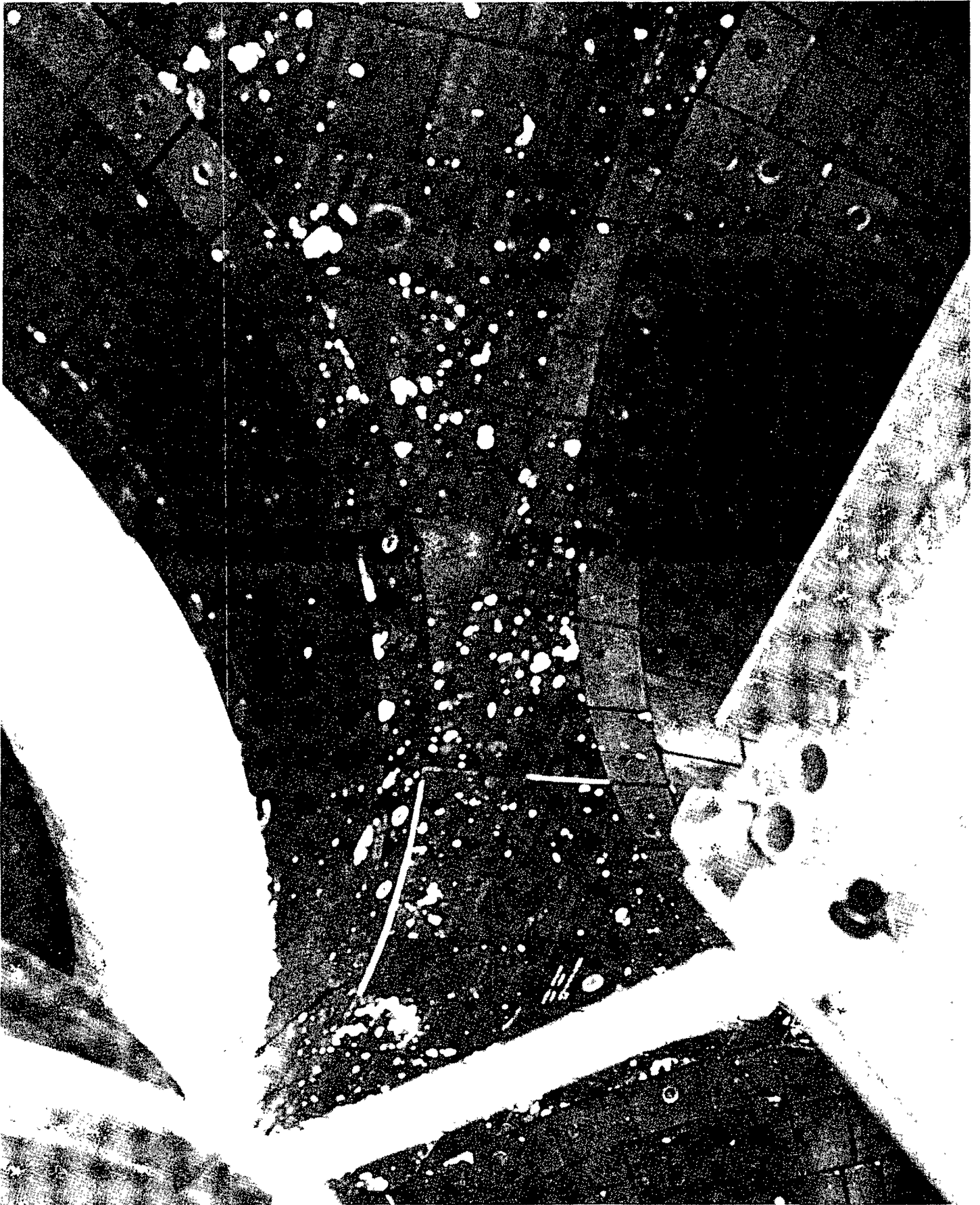
TYPICAL DAMAGE TO TILES ON ORBITER AFT HEAT SHIELD
