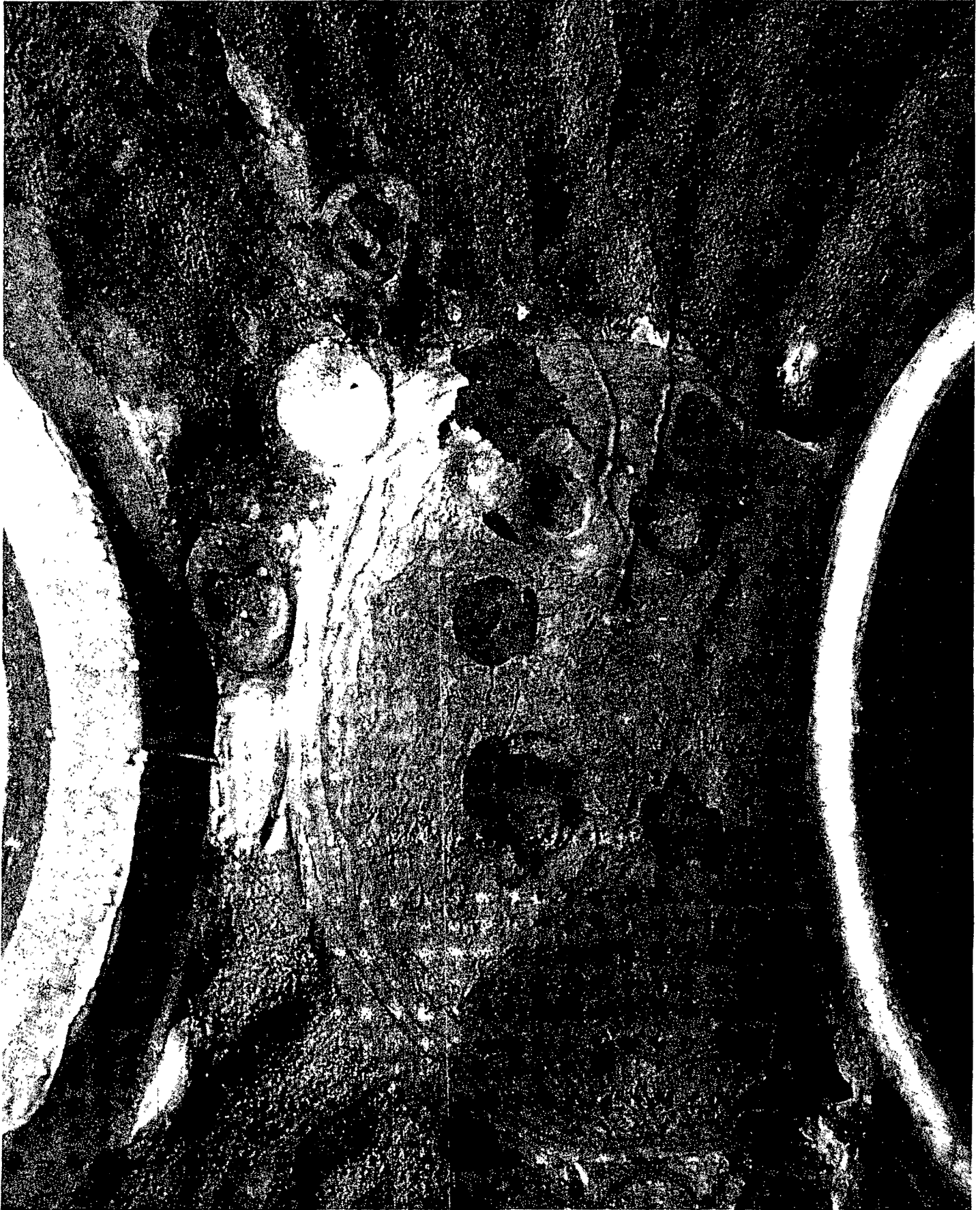
FROST LINES APPEAR ON LH2 TANK AFT DOME VENDOR REPAIRS. CONDENSATE DRIPS FROM MANHOLE COVERS AND AFT DOME APEX.
