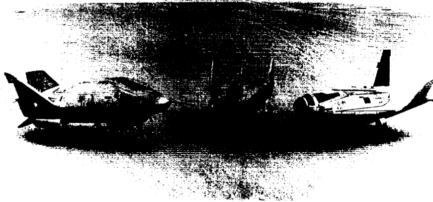
Three lifting body configurations grouped on the dry lake bed at Flight Research Center. Left to right: the X-24, M-2, and HL-10.
