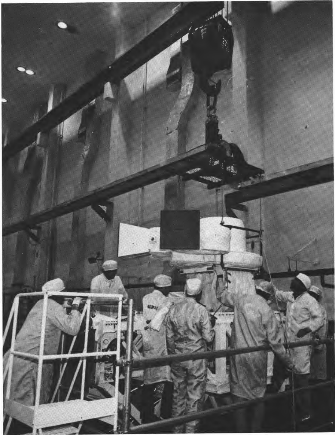
Figure 2-2.- The LFC/SCA, shown being placed on the MPES by KSC integration personnel. (NASA photo S85-26826.)
