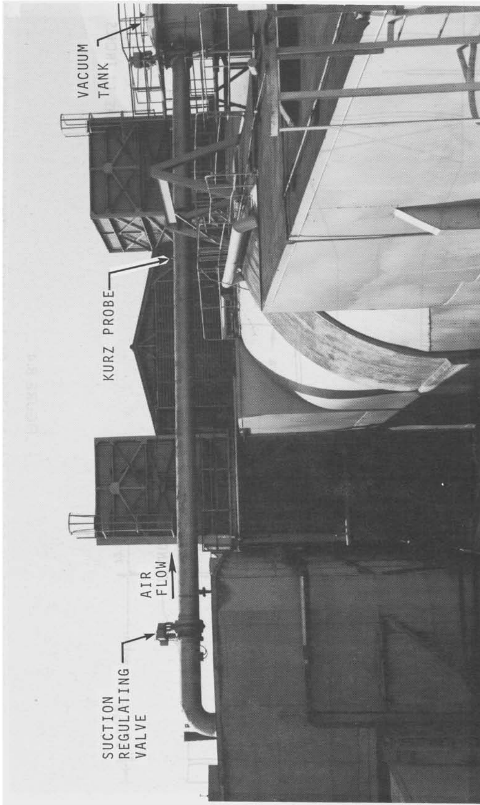
FIGURE B.5 VACUUM TANK AND 24 INCH ID DUCT OF THE NASA SUCTION SYSTEM.
