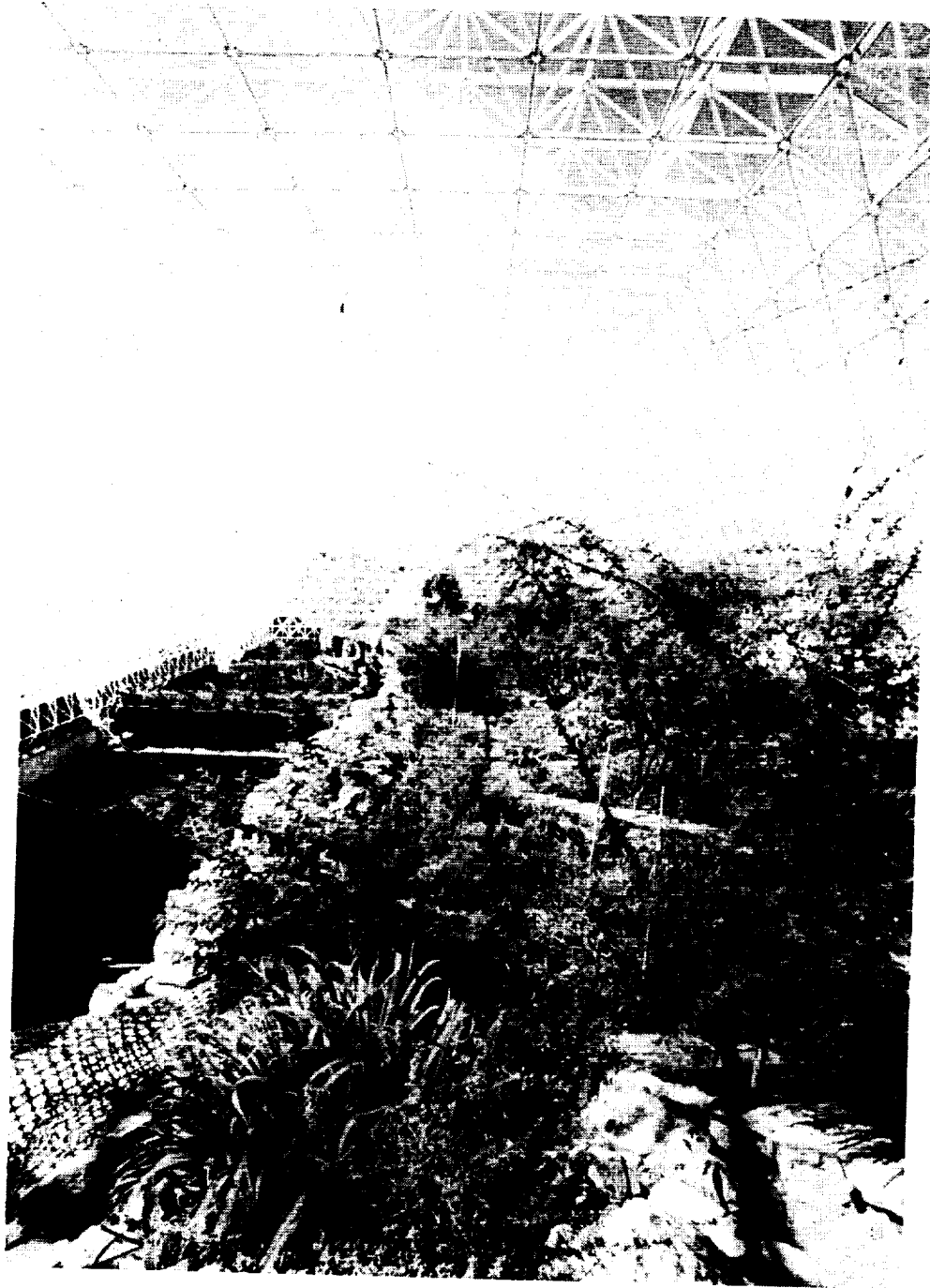
Figure 8. Biosphere 2 wilderness biomes under construction, interior view. Savannah at right; marsh biome upper left, marine biome lower left.
