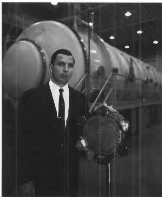
Harold R. Kaufman with his electron bombardment ion thruster.
