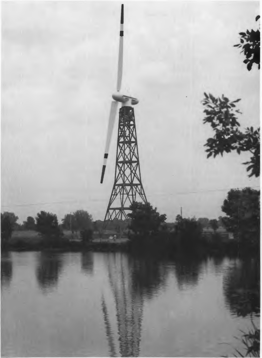
100-kilowatt wind turbine at Plum Brook.
