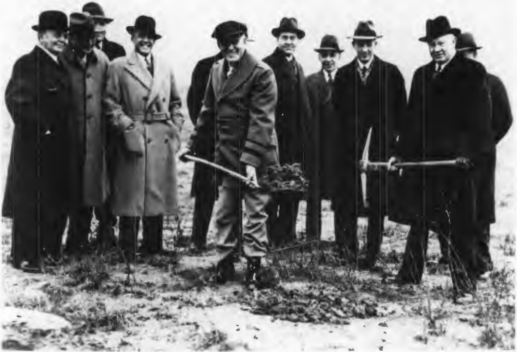
The frozen ground required both pick and shovel at the ground-breaking ceremony for the new Aircraft Engine Research Laboratory next to the Cleveland Municipal Airport. Left to right in the foreground are William R. Hopkins, former city manager who developed the airport; John Berry, Airport Commissioner; Frederick C. Crawford, President of the Cleveland Chamber of Commerce; General George Brett, Edward Warner, and Captain Sidney Kraus of the NACA Main Committee; Edward Blythin, Mayor of Cleveland; and George W. Lewis, NACA Director of Aeronautical Research.
