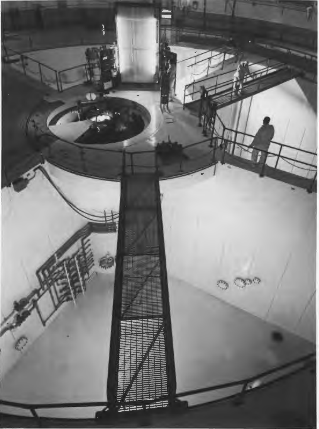
Water-filled quadrants surrounding the Plum Brook nuclear reactor, 1961.
