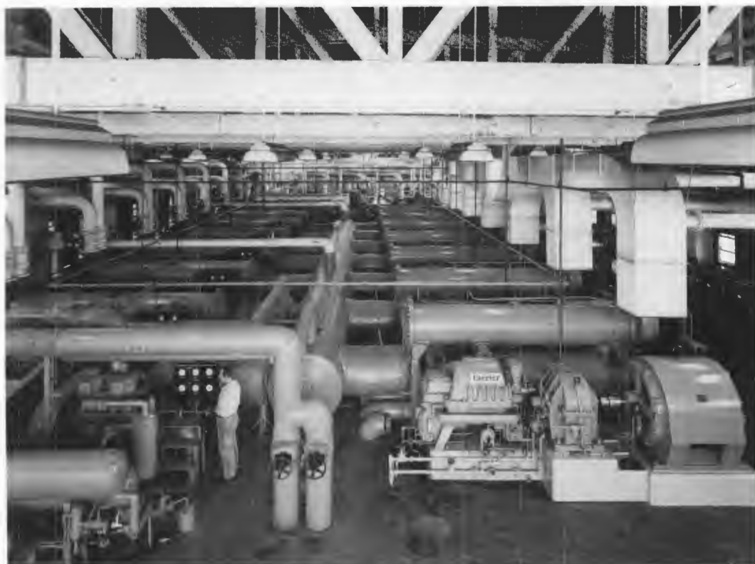
Top: The Altitude Wind Tunnel urgently needed for full-scale engine testing. Bottom: Innovative Carrier compressors chill the tunnel's airstream.
