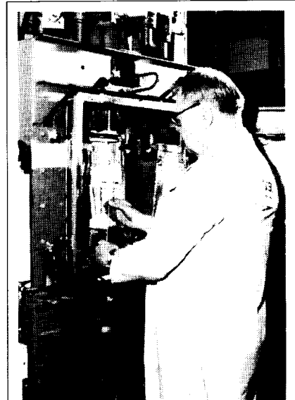
One of three furnaces in Multiparameter Mission Simulation Facility used to evaluate ORCC composite materials. 1-89-00781
