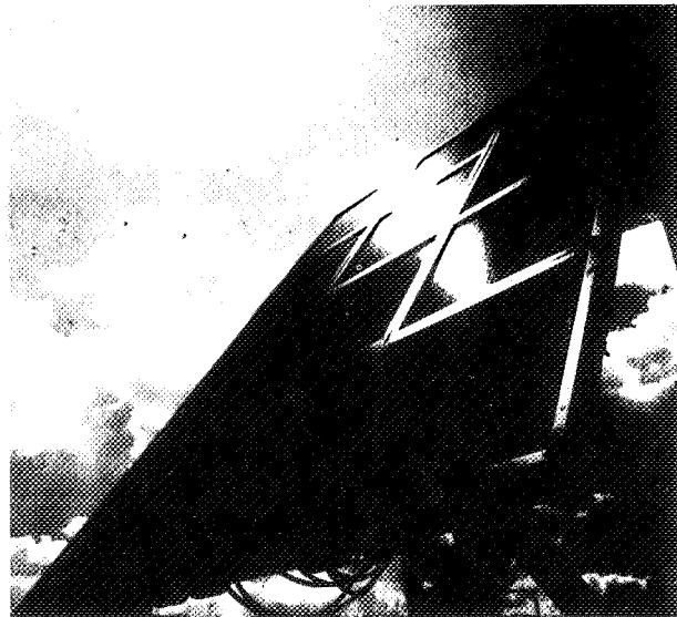
Figure 11. A 54 W thin-film CdTe array for water pumping deployed by BP Solar in Saudi Arabia.
