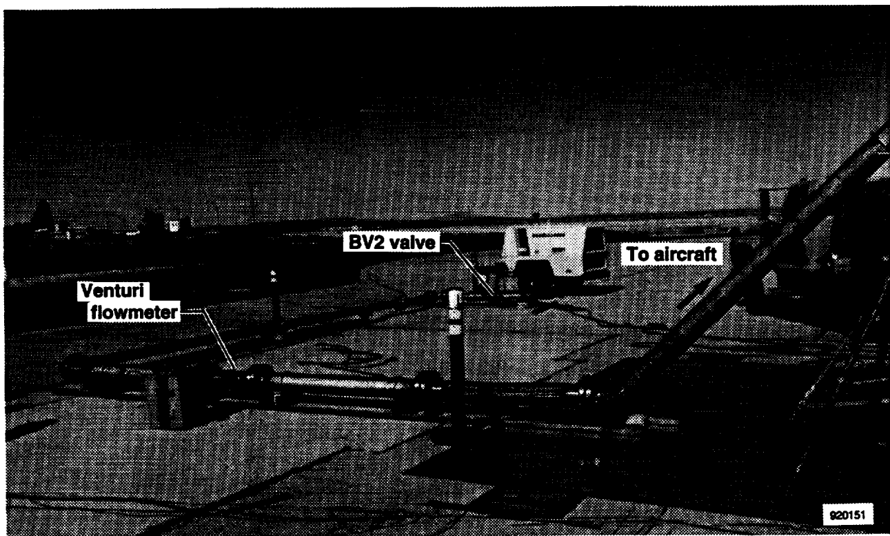
Fig. 6. Excess bleed air system ducting, bleed flow dump section.
