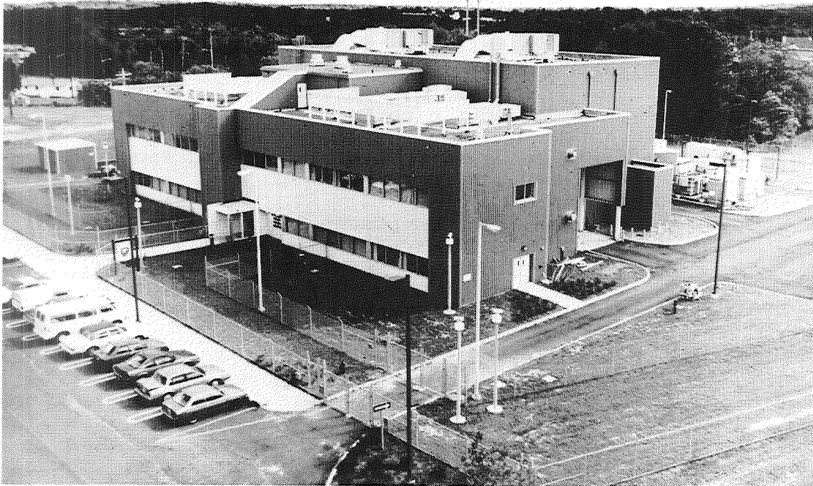
Figure 1: The U.S. Army Pulse Power Center at Fort Monmouth, NJ
