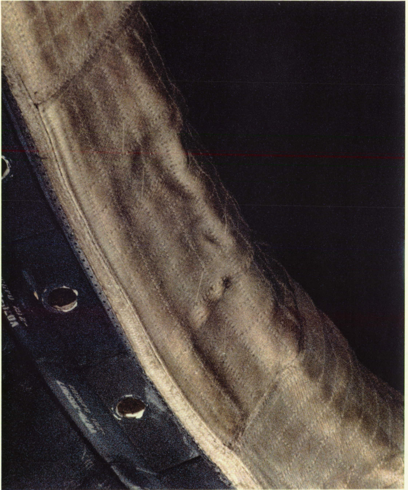
The Orbiter SSME #2 Dome Mounted Heat Shield (DMHS) closeout blanket appeared to be scorched and discolored
