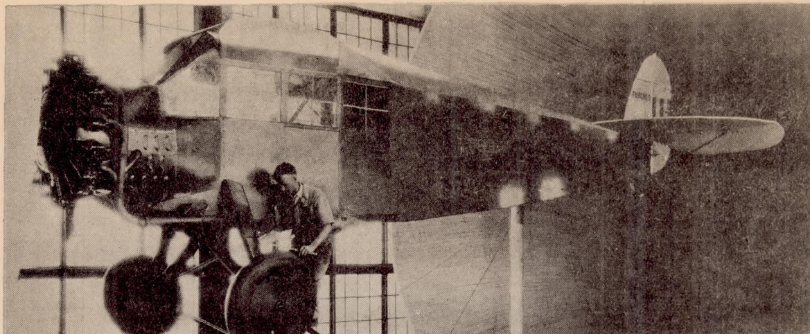
Fig. 9. TURTLEBACK AND WING ROOT FAIRINGS ADDED.
