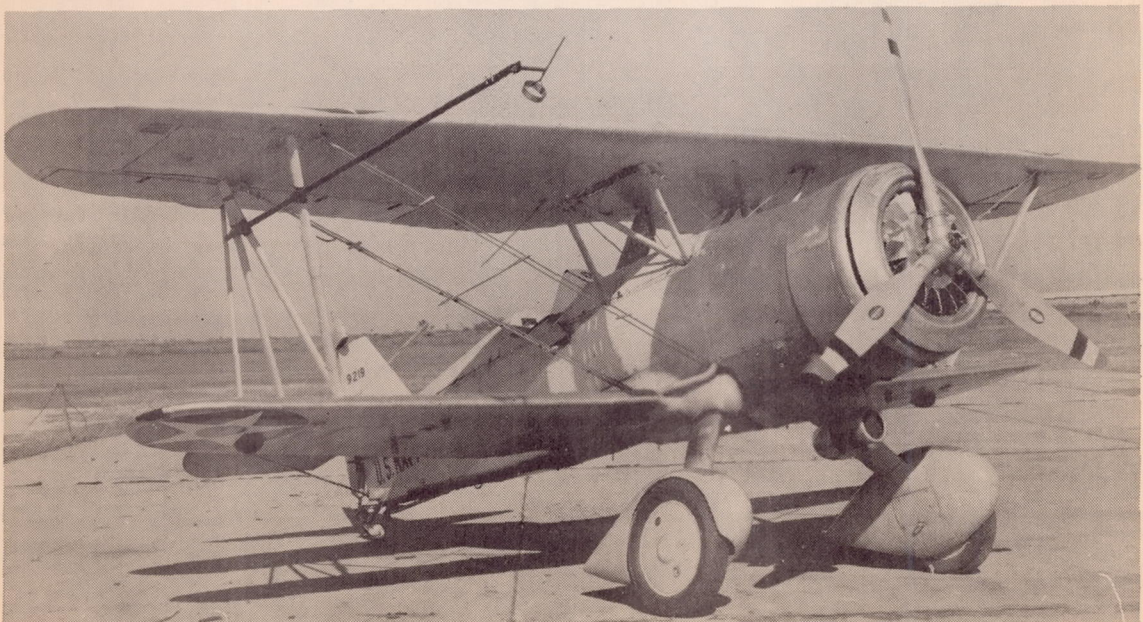
Figure 7.- Nose-slot cowling 3-F with countervanes in place on the BFC-1 airplane.
