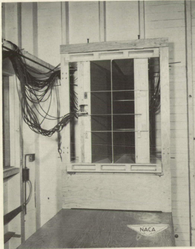
Figure 11.- Diffuser with central partition.
