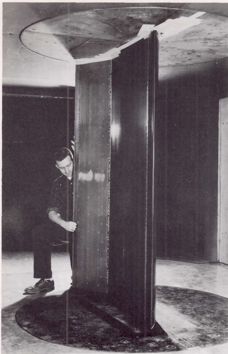
Figure 1.- The NACA 0006 airfoil mounted in the Ames 7- by 10-foot wind tunnel.
