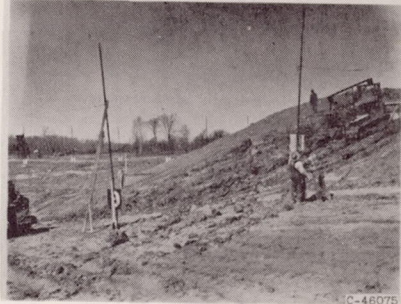
(b) Earthen mound that airplane struck after landing gear was removed.
