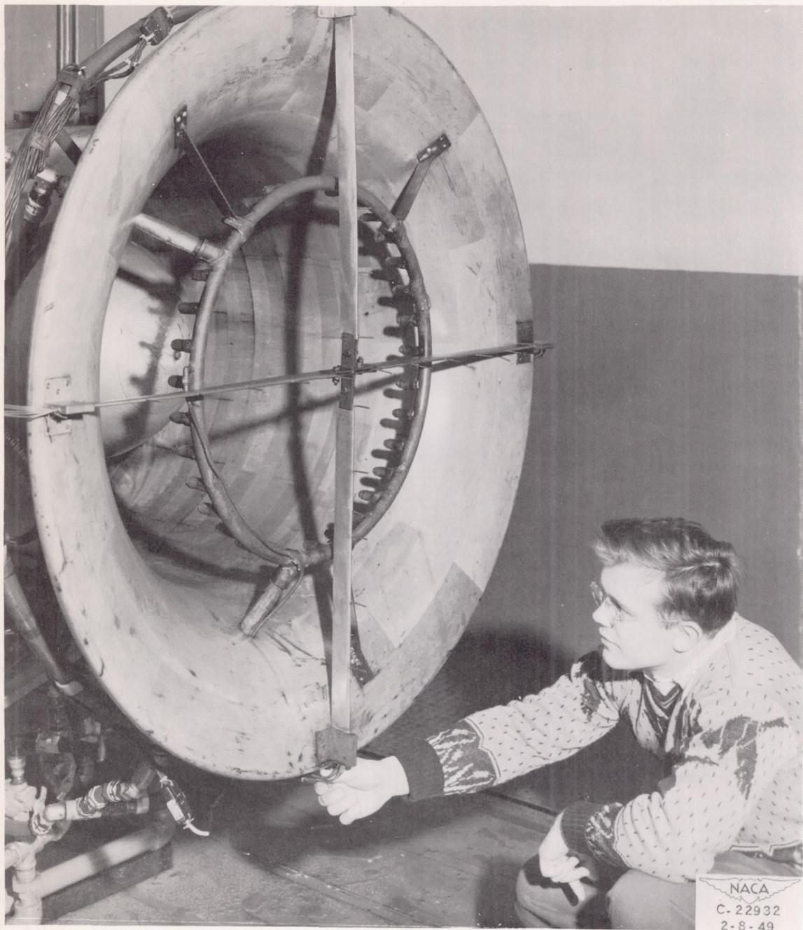
Figure 2. - Engine inlet cowling showing installation of atomizing nozzles.
