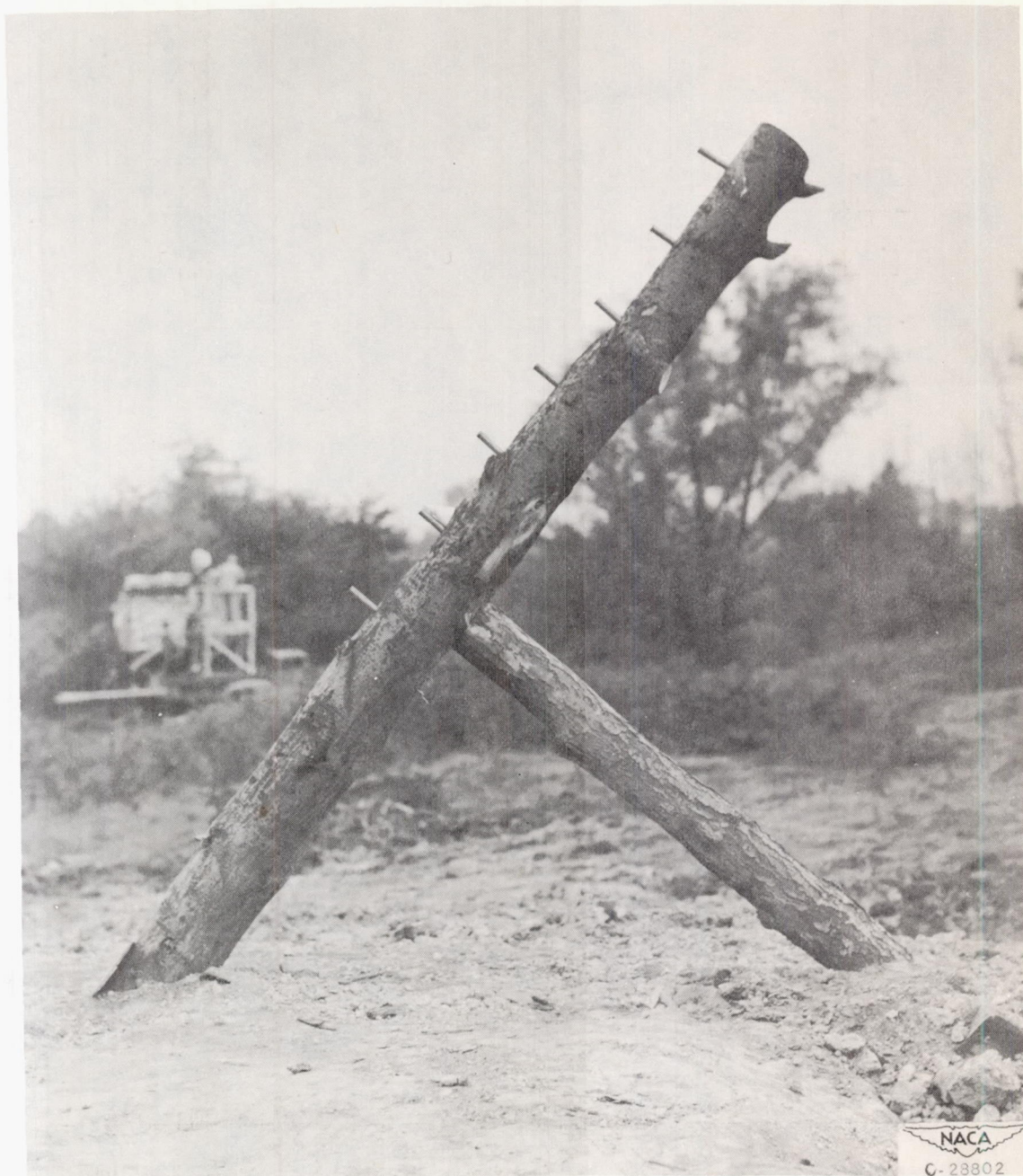
Figure 12. - Close-up of pole barrier showing steel spikes.
