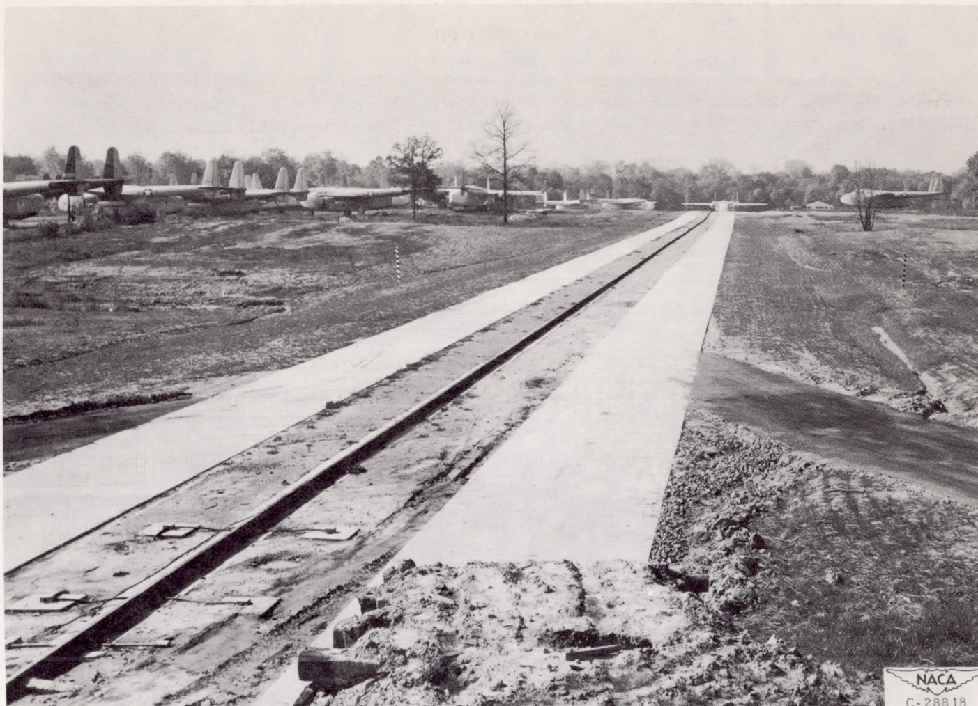
Figure 6. - Runway and center rail for guiding airplane to crash barrier.
