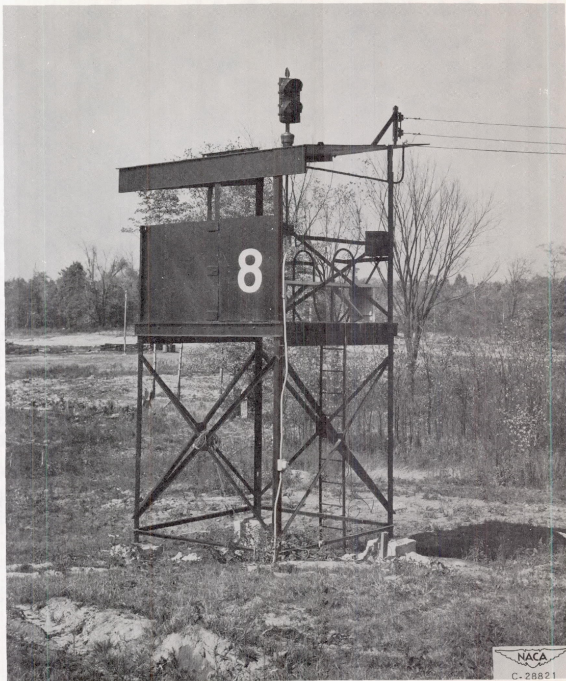
Figure 18. - Typical camera platform installation in crash area.
