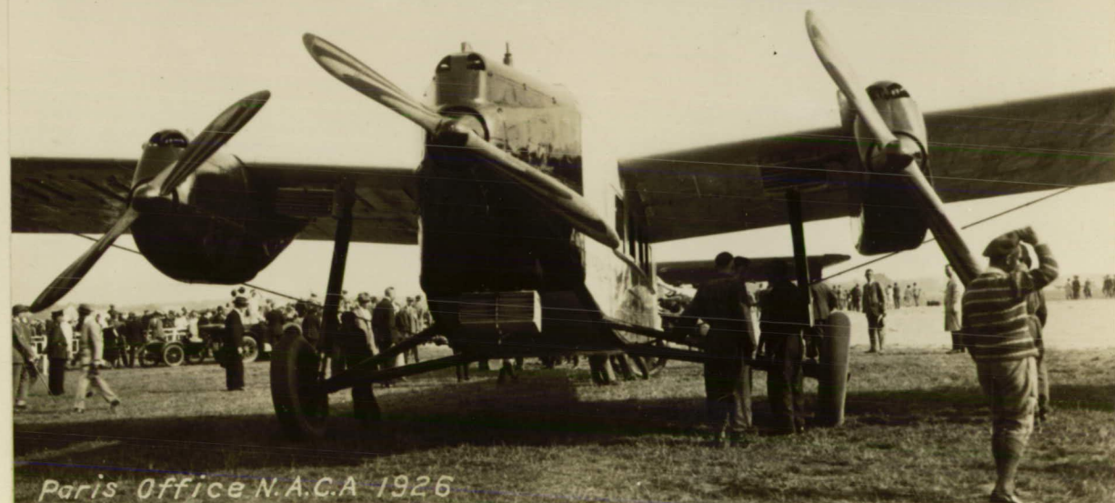
Figs.2,3 & 4 Rhorbach - Roland Ro VIII commercial airplane with three 230 HP. B.M.W. engines.
