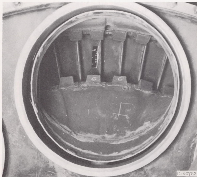
(b) Least damaged sector.
