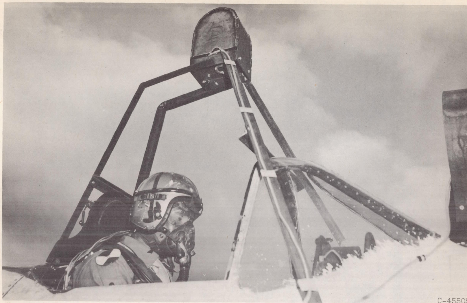
Figure 5. - Concluded. Location of cameras installed on airplane to photograph dummy's action during crash.
