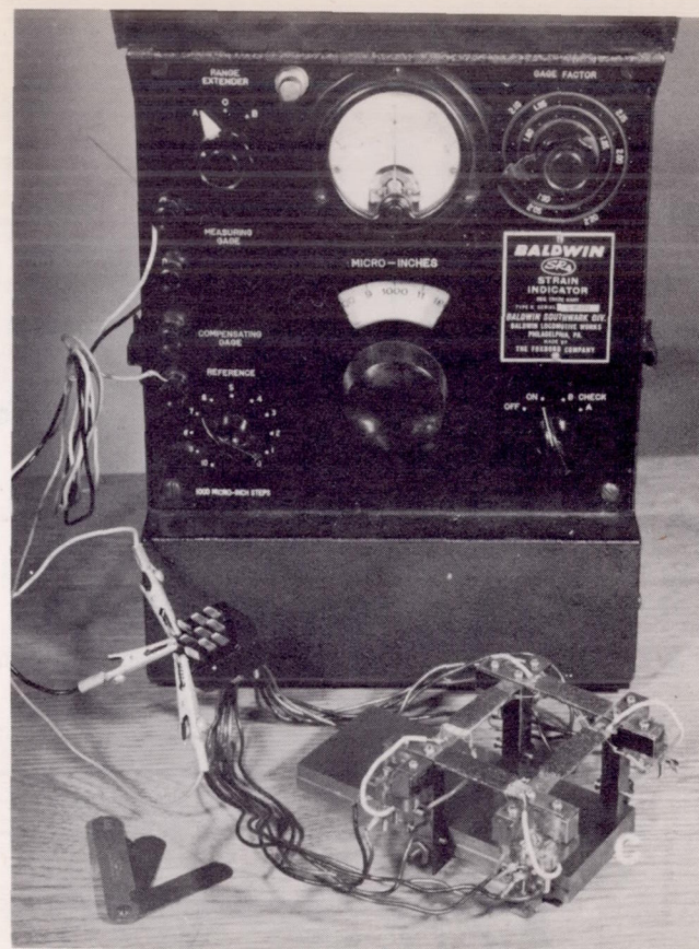
(b) Device for calibrating clip gage.
