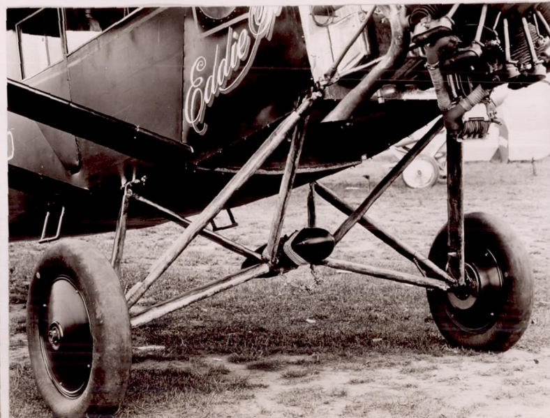
Fig. 4 Split type landing gear. Note the brake cables which emerge from streamline fairings at lower end.
