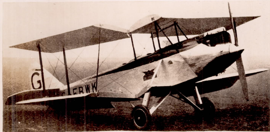
Fig. 6 View of the Avro "Avian III" showing port wings spread and star- board wings folded, to illustrate how landing gear wheels move back when the wings are folded. The telescopic jury struts fold flat against the top wing when in flight.
