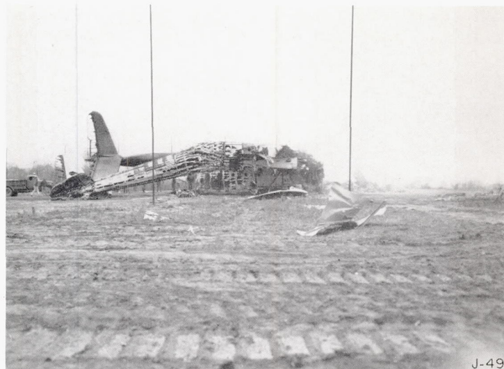
FIGURE 64.—Structural collapse due to melting and burning of skin and structural members.
