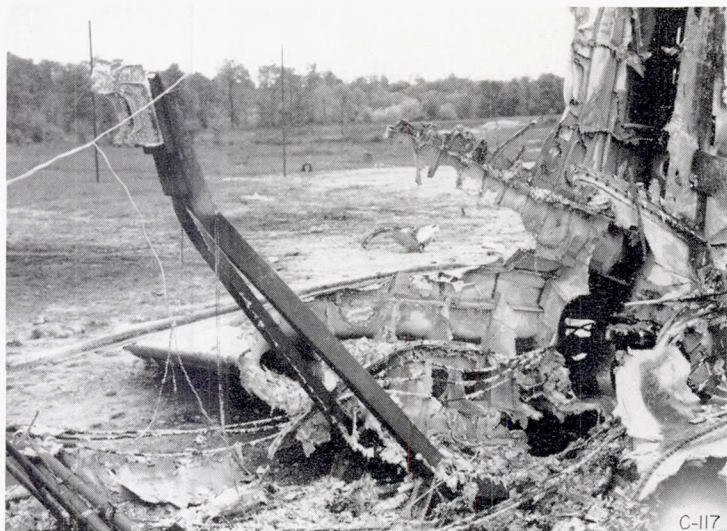
FIGURE 63.—Structural elements melted in a typical crash fire.
