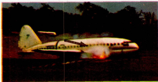
(c) First oil fire outside of nacelle; 3.42 seconds after initial impact. Airplane speed, 2 feet per second.
