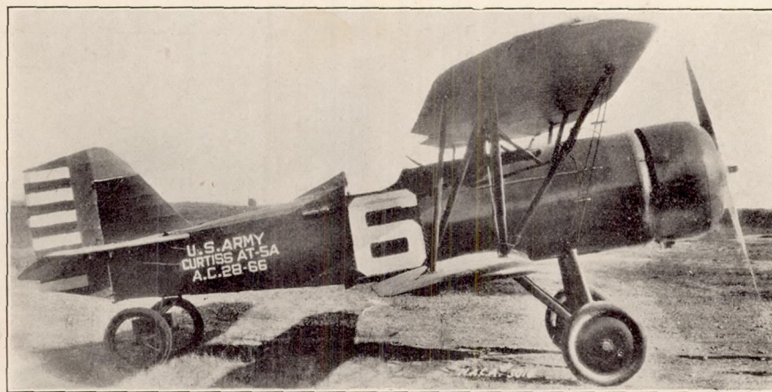
FIGURES 34, 35.—Curtiss A T-5 airplane with No. 10 cowling
