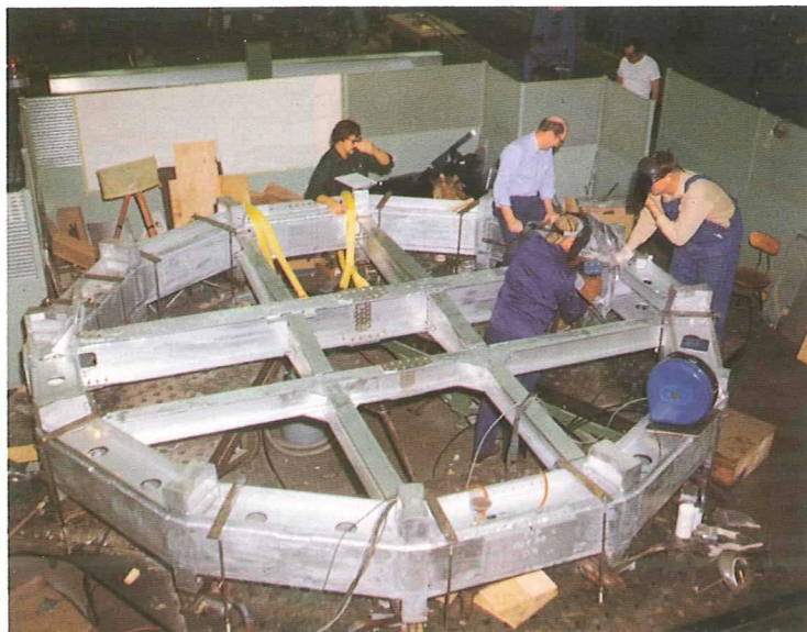
Fabricating LDEF's center ring frame
