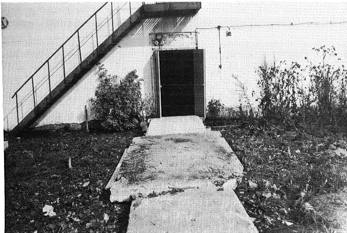
FIGURE 9 RUNWAY FROM PAVED ROAD TO BUILDING
