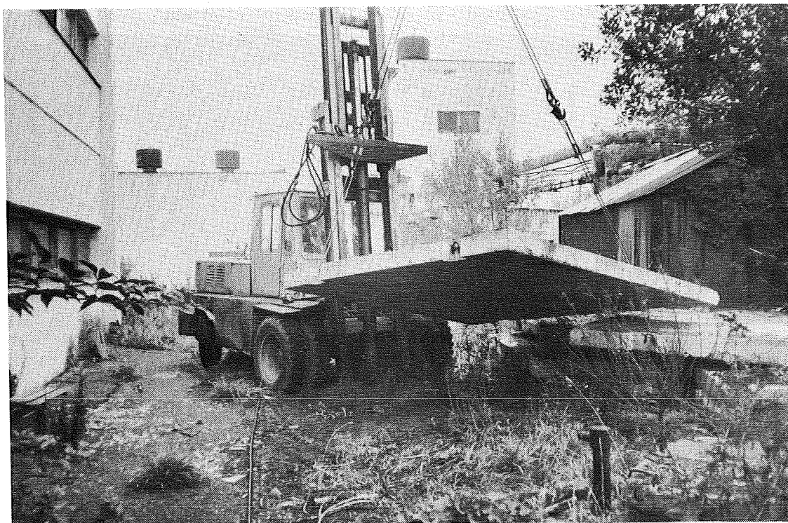
FIGURE 10 TRANSPORTING SLABS TO RUNWAY AND COMPRESSOR SITES
